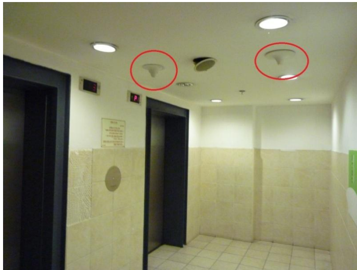
An example of picocell providing indoor coverage
